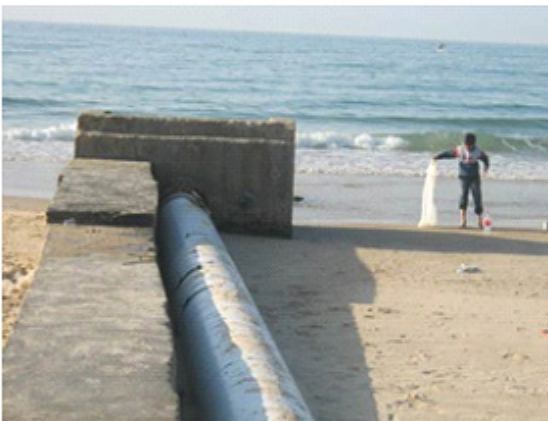
The Brine Outlet of the DeirEl-Balah seawater RO Desalination Plant
