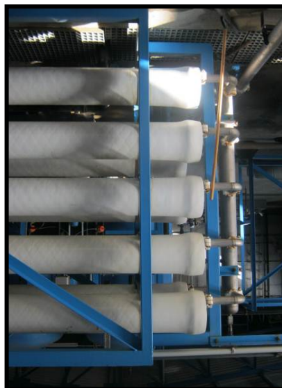
Figure 14: Deir El Balah desalination plant: The entry (Right) and the RO filter membranes (Left)
